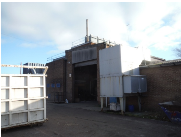
Photograph 5 – View of the HVAC unit adjacent to the former furniture works
