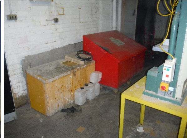
Photograph 8 – View of chemical store to the southern part of the warehouse
