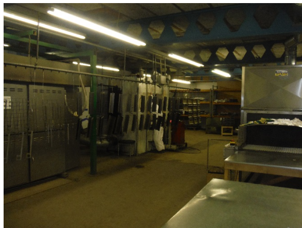
Photograph 9 – View of metal works
