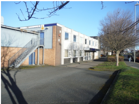
Photograph 1 – View of the furniture factory, looking northwest.
