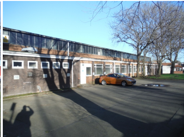
Photograph 2 – View of the furniture factory, looking northwest.
