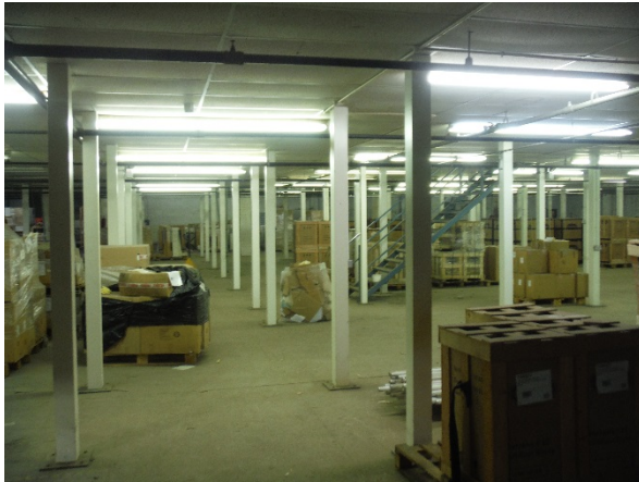
Photograph 3 – View of the storage area with mezzanine level.
